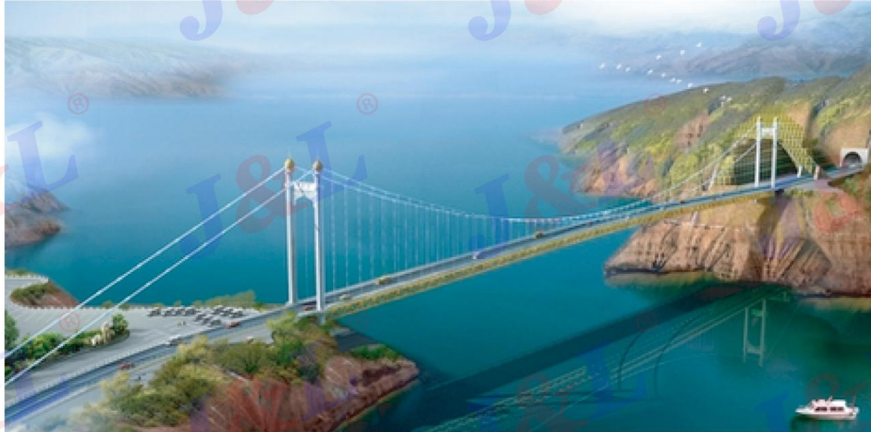
LIUJIAZIA YELLOW RIVER BRIDGE
