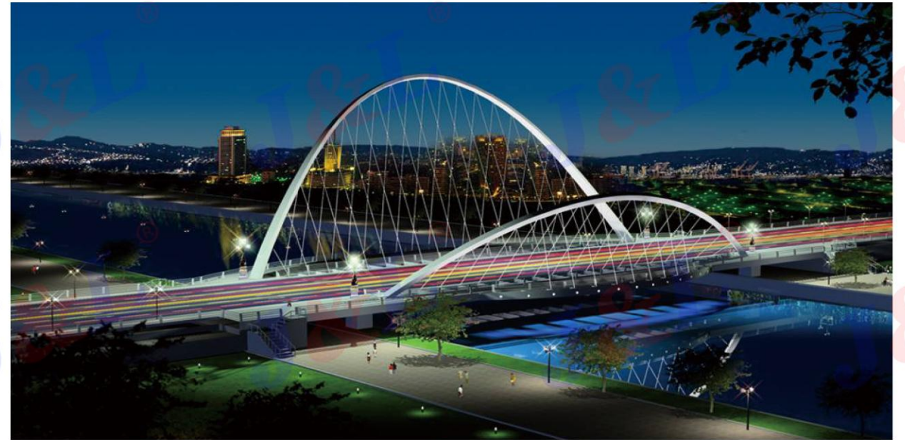
TIANJIN DAGU BRIDGE
