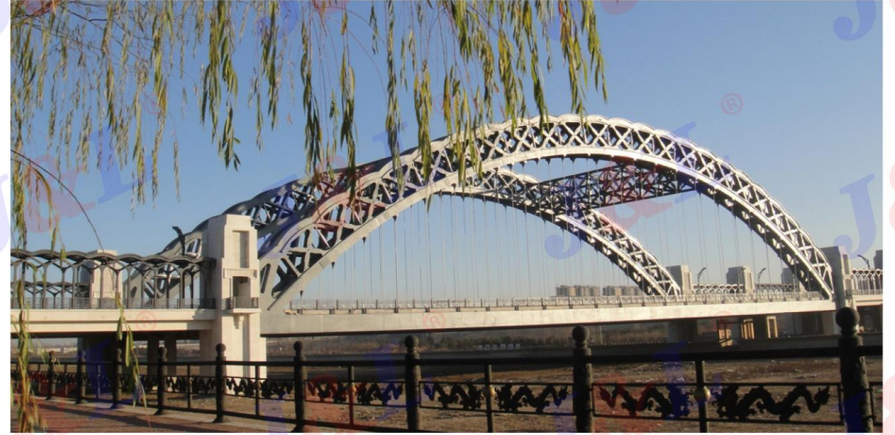
DATONG PINGCHENGJIE YUHE BRIDGE
