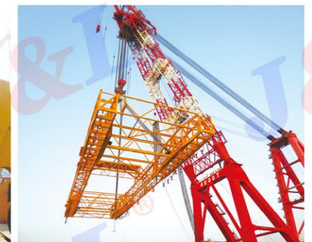
3660T WORKING LOAD BRIDGE FLOOR LIFTING APPLIANCE FOR GANGZHUAO BRIDGE
