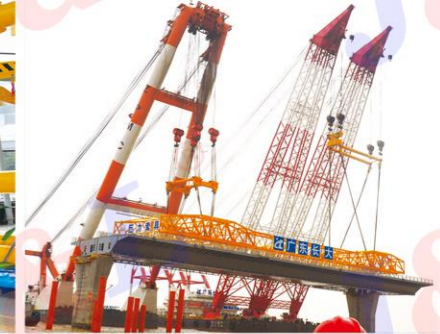
3400T WORKING LOAD BRIDGE FLOOR LIFTING APPLIANCE FOR GANGZHUAO CHANGDA SECTION
