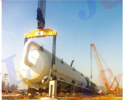
LIFTING APPLIANCE FOR LARGE PETROCHEMICAL EQUIPMENT
